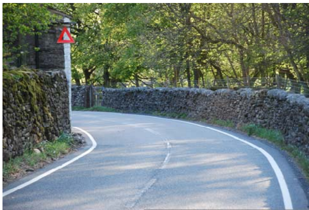
H. Road is less than 3.85m wide here. The white line has been scrubbed off but there is no warning that the road is basically a single track width other than a 'road narrows' sign similar to those placed in numerous other sections of the road.
